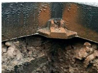
Closer inspection determined a lack of support under the ironwork in critical functional areas.
