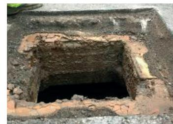
Evidence of the incorrect type and amount of material needed to ensure a durable installation.
