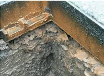
The supporting structure and chamber were in poor condition, it was also evident that the bedding materials used had failed.
